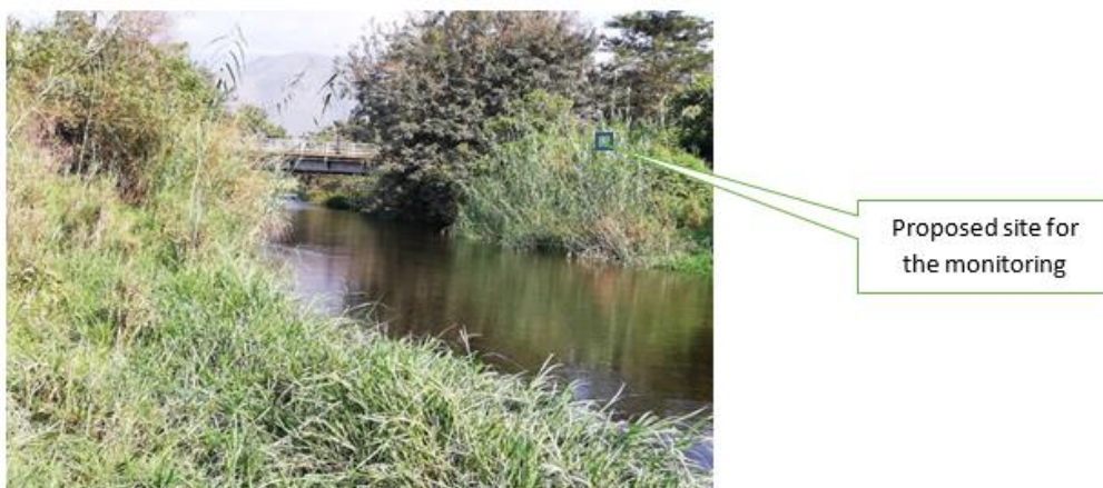
Photo 5: Showing Nyamwamba Bridge and the surrounding flora near the site
