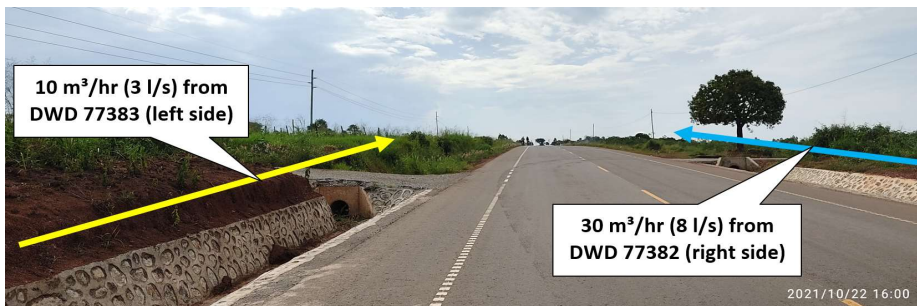
Figure 5-15: Transmission mains from both boreholes moving along the Kigumba – Masindi road
