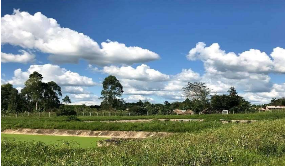
Figure 7-3: Waste Stabilization Ponds at Kiryandongo Hospital
