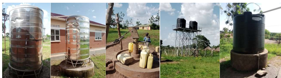
Figure 5-69: RWHTs, Borehole, Storage tanks at Apodorwa HC III with support from OPM/DRDIP/ World Bank
