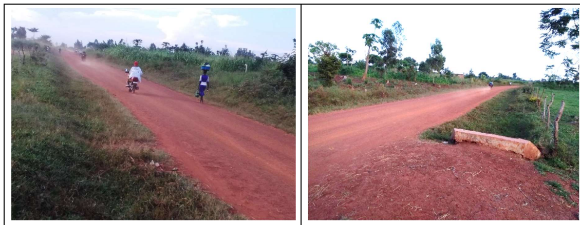
Figure 0-36: Dust emission caused by Bodaboda traffic along Mutunda – Diima road
