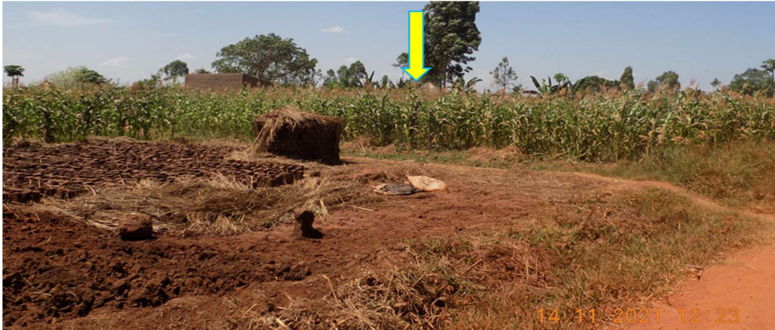
Figure 0-9: Existing environment and access of Alero B reservoir tank
