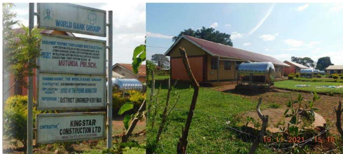
Figure 0-70: Steel water tanks at Mutunda primary School
