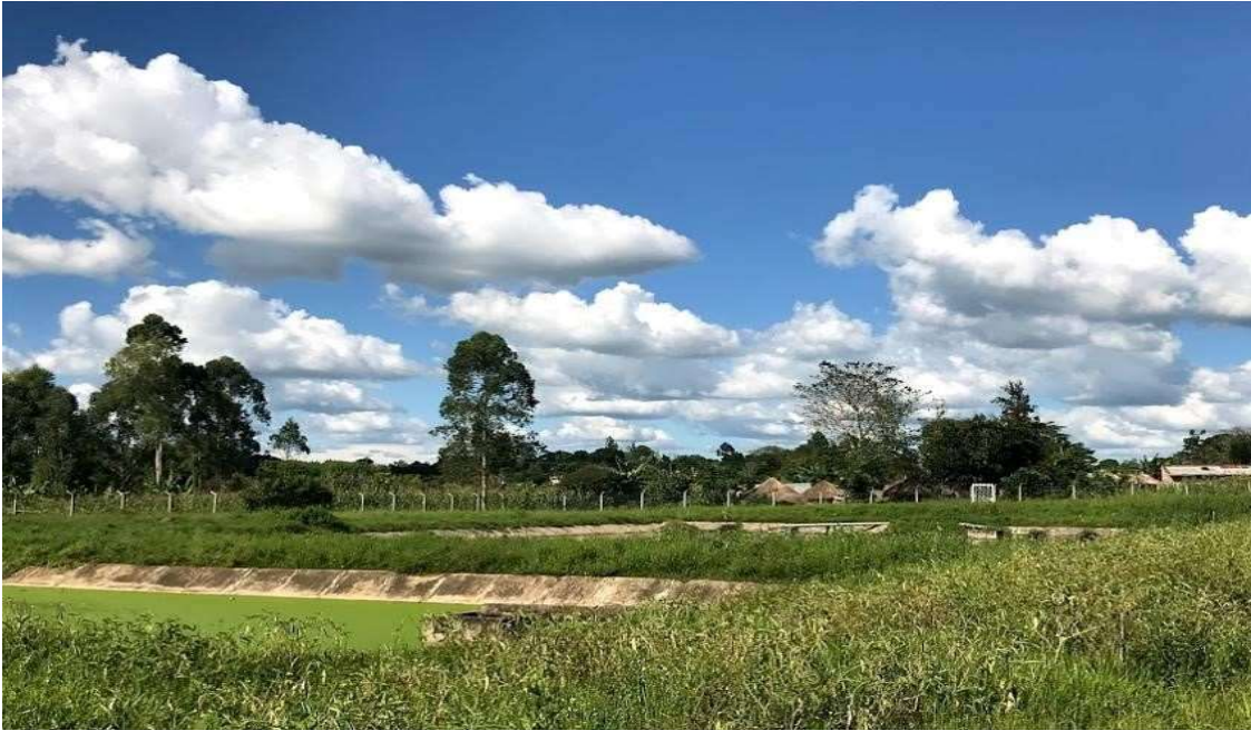
Figure 0-3: Waste Stabilization Ponds at Kiryandongo Hospital
