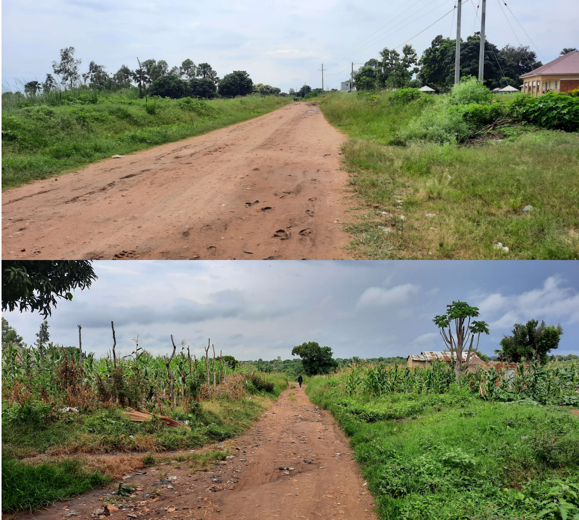
Plate 5-3: Existing Road Condition around the project site
