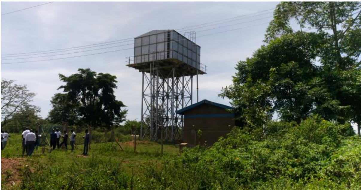
Photo 2-5: Proposed and Existing Reservoir location at Tirinyi
