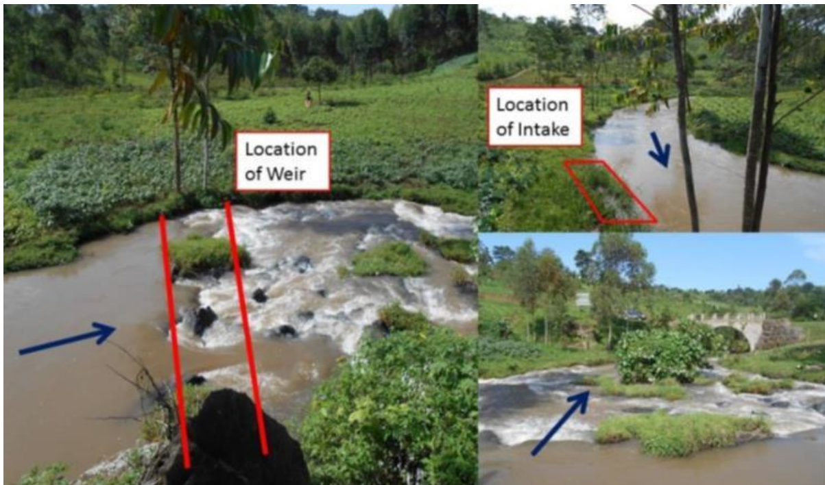
Photo 2-1: Proposed location of intake and weir (36N 640429 122846)
