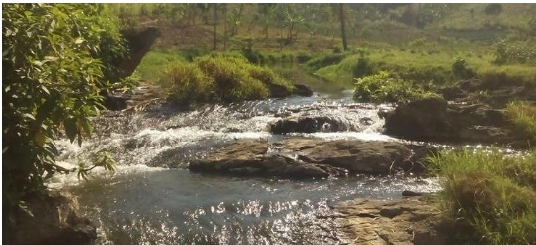
Photo 5-2: Proposed site for the intake works on River Namatala
