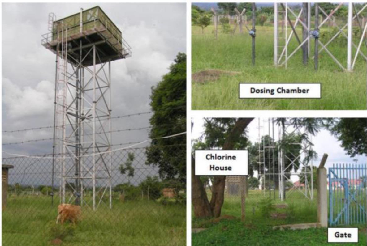
Photo 2-2: Existing reservoir structures at Budaka (36N 607206 112784)
