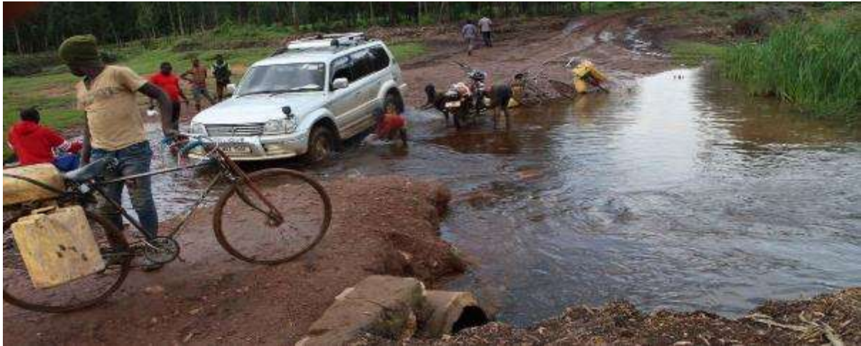
Figure 4-65: Poor road and river stream used as water sources in the irrigable area at237333, 9895668
