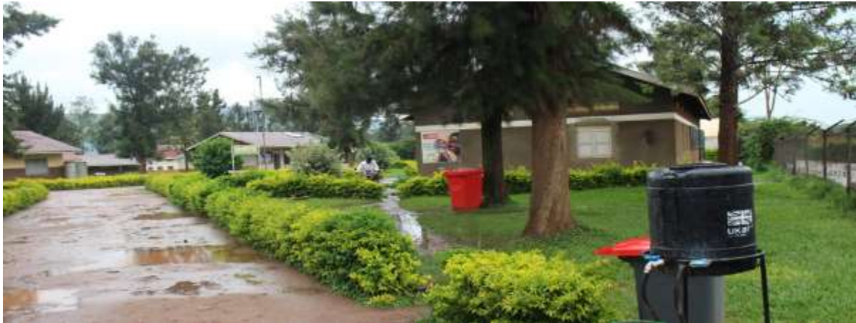
Figure 4-76: Kabuyanda Health Centre IV in Kabuyanda TC (irrigable area E235650, N9895152)
