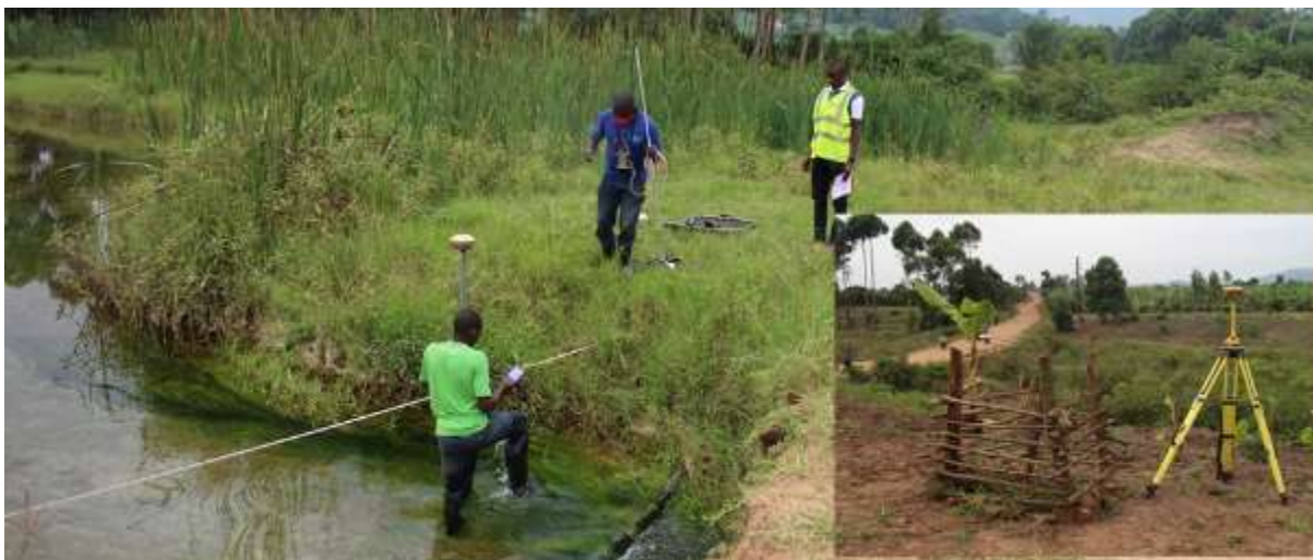
Figure 3-5: Picking the dry and wet profile cross-sections of Mishumba using an RTK machine
