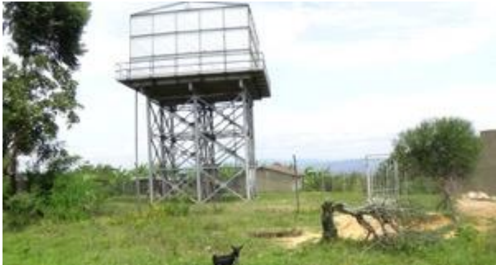
Plate 4: Location of the Bwoma Reservoir site.
