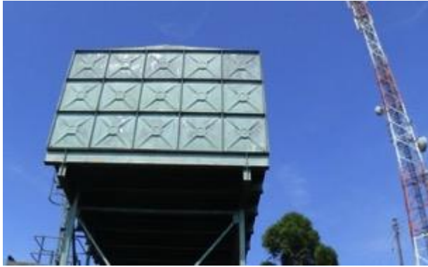
An existing water reservoir
