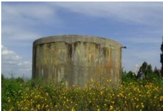
A concrete water reservoir on the site
