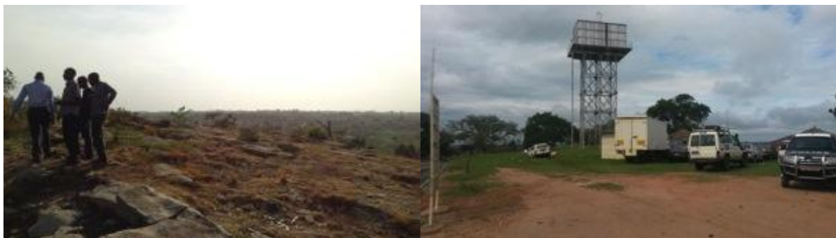
Plate 16: Location for Teremunga reservoir (left) and Appa Reservoir (right).
