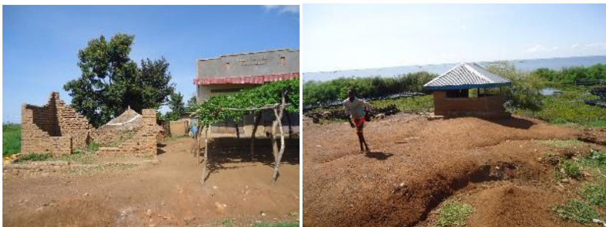
Plate 7.2: Some of the structures that will be affected at Biko landing site where the water treatment plant will be constructed.
