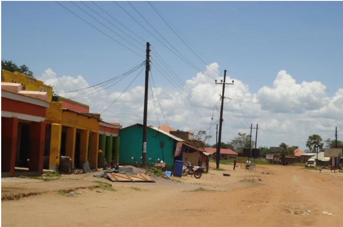
Figure 4-13 : Power distribution lines in Namasale town
