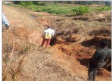
Extensive erosion of the downstream embankment and foot-slopes of a small dam
