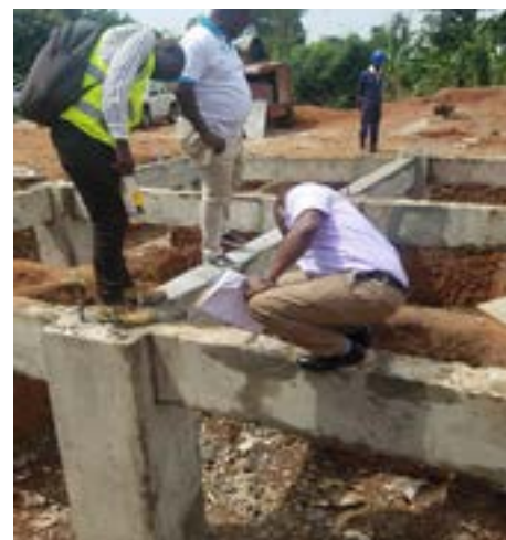
Recent Compliance Audit
