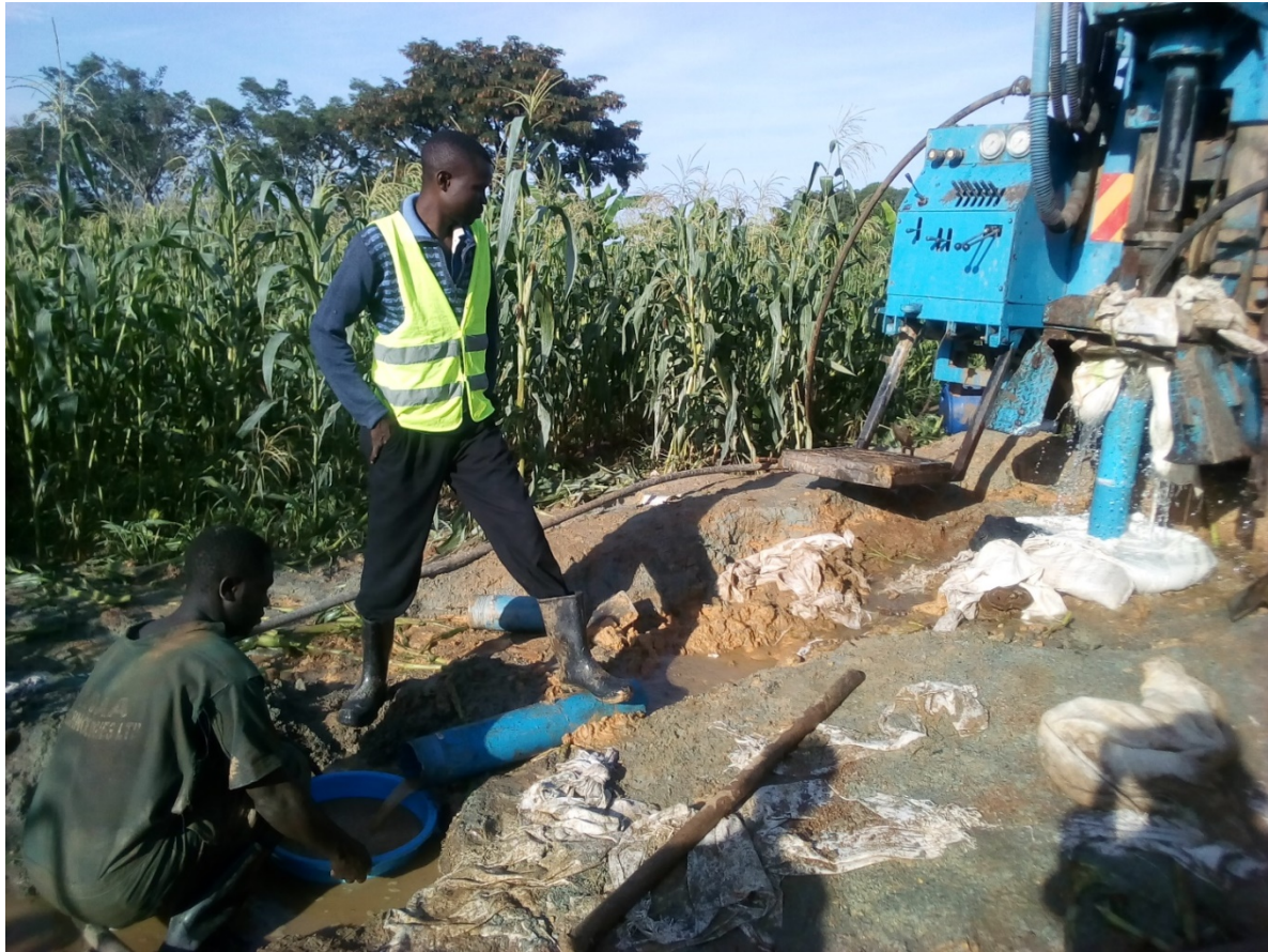
Airlift yield estimation during drilling
