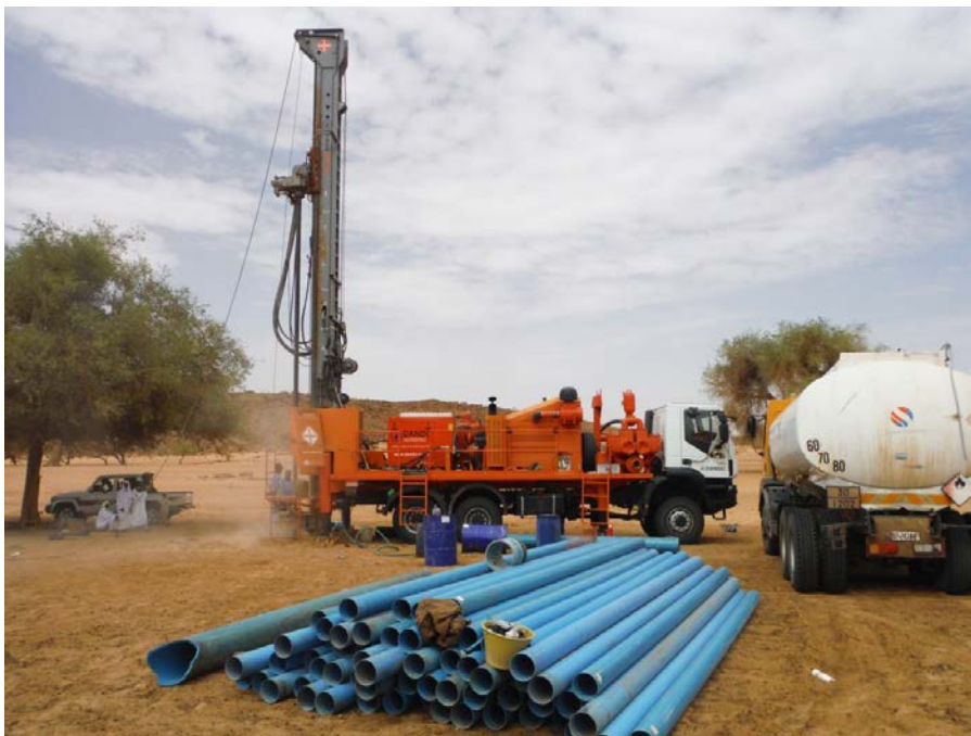
Equipment and materials for borehole construction
