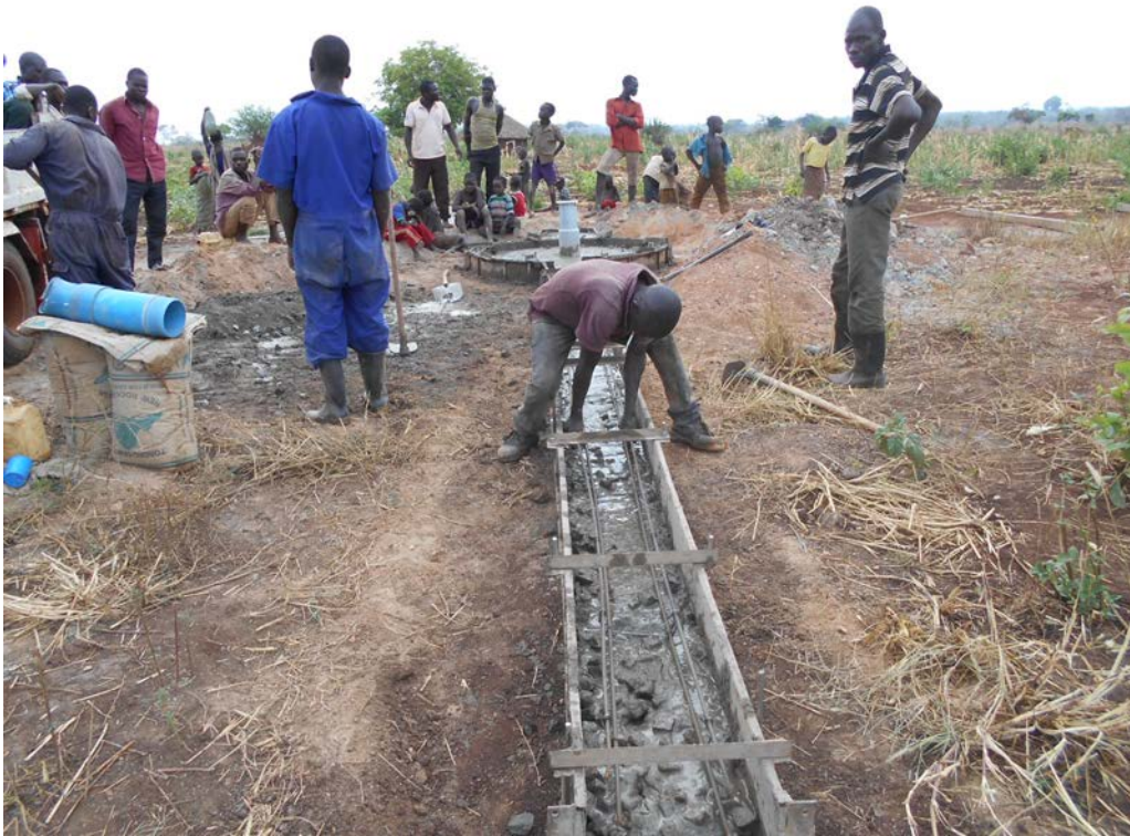
Demonstration of borehole casting
