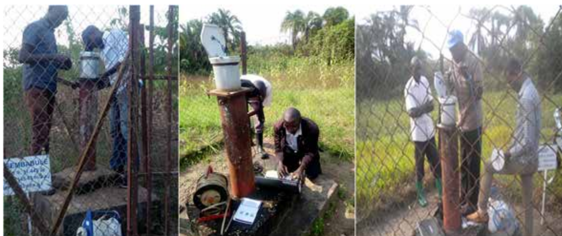
Installation of Telemetric Equipment at one of groundwater monitoring station
