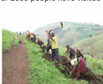
Construction of earth bunds
