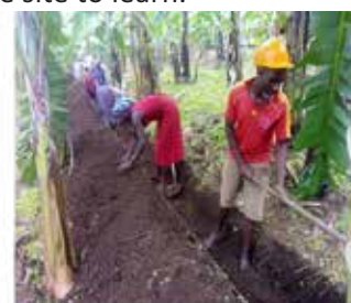
Construction of infiltration trenches
