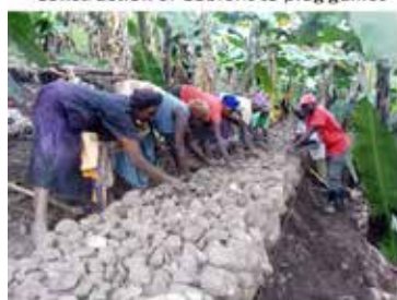
Construction of stone bunds
