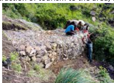
Construction of Gabions to plug gullies
