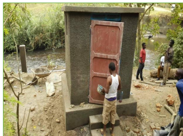
Construction of the river gauging station
