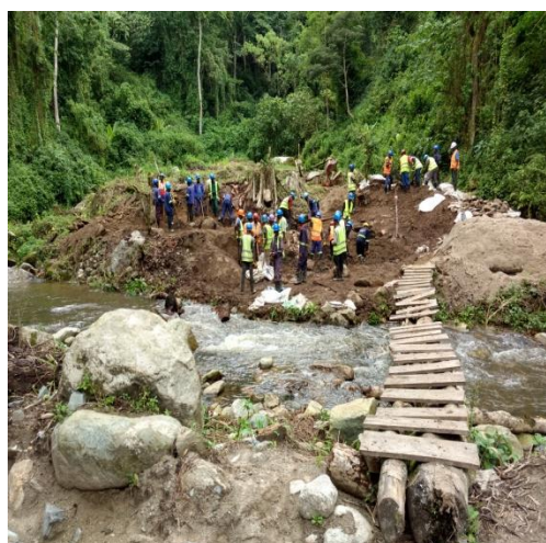
Excavation at the project site
