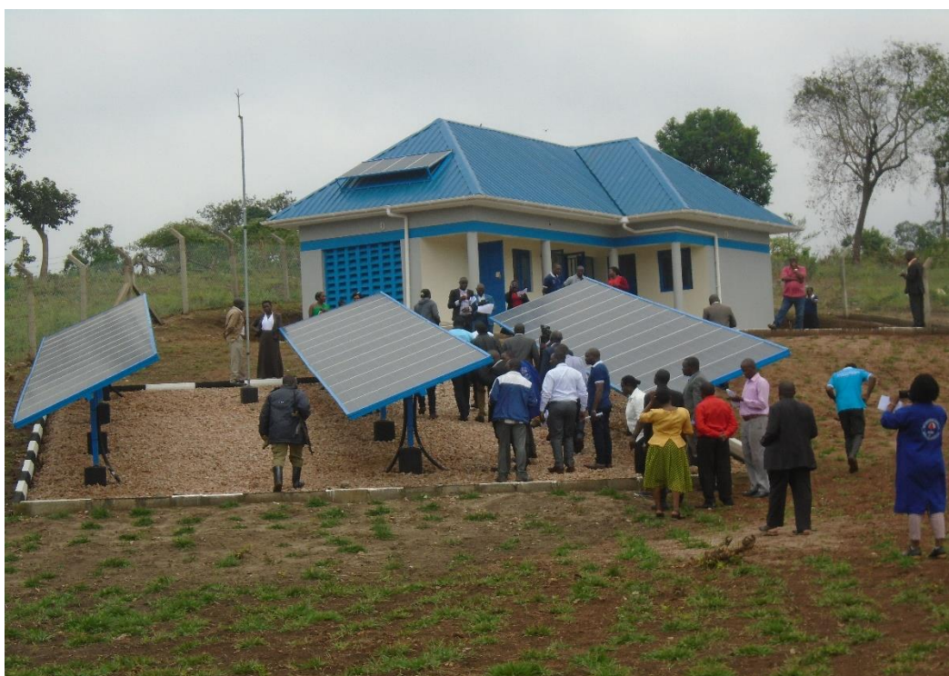
Solar Powered Piped Water Supply and Sanitation System in Kibaale District
