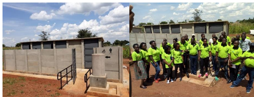
Completed sanitation facility at Kamdini primary school in Oyam District
