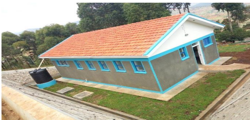
Gender Segregated Water Borne Toilet with 10 stances of which two stances are for disabled and bathroom for girls constructed at Tulel Secondary School in Bukwo District
