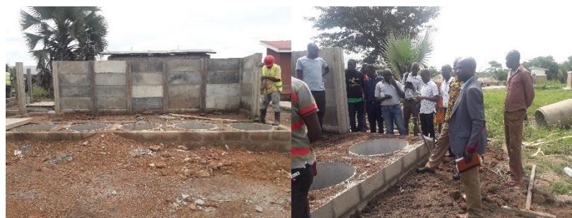
Construction of the super structure in Alukot Primary School in Oyam District
