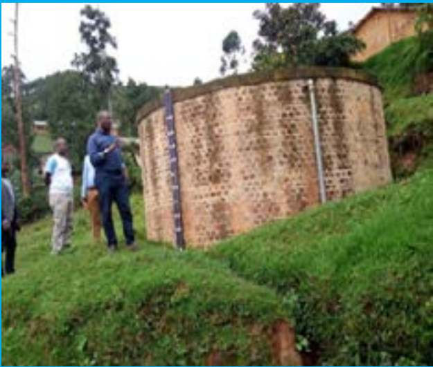
Reservoir at Katuna WSS
