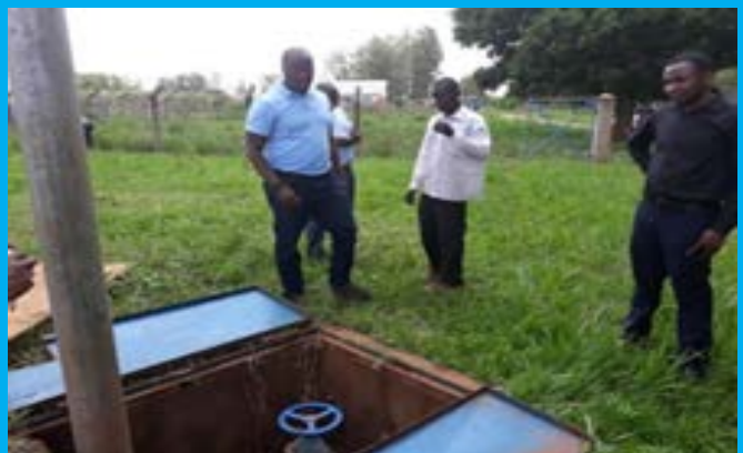
Ag. Asst. commissioner observing the faulty bulky meter at Minakulu
