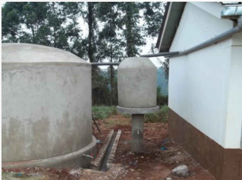
Figure 9: Large capacity first flush device with washout valve for easy operation
