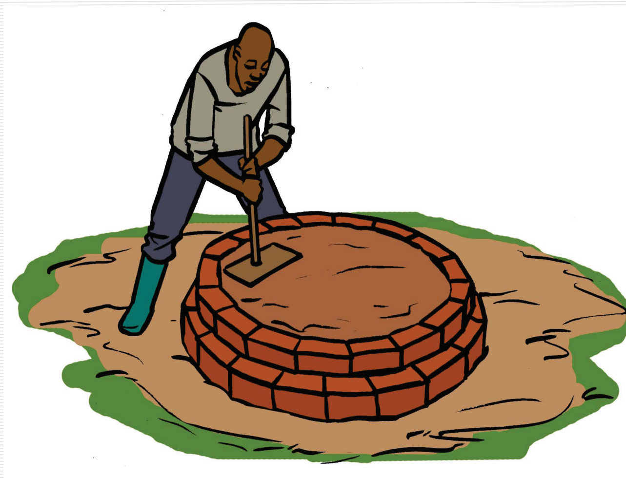
Figure 45: Lay line of bricks up to 1m and compact the earth
