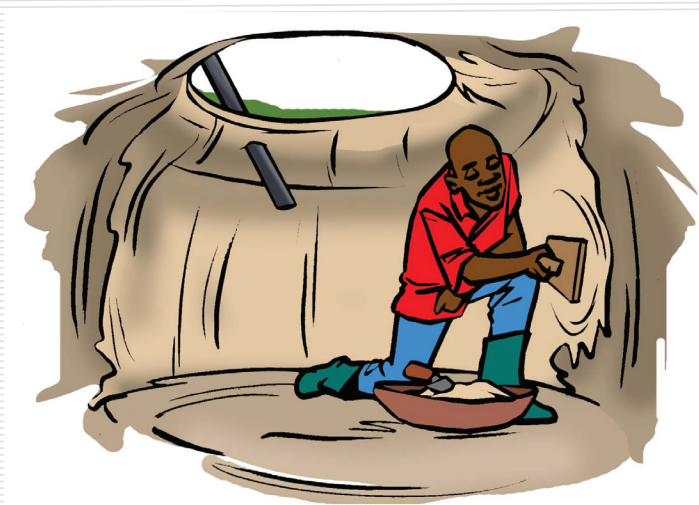
Figure 43: Applying water proof cement
