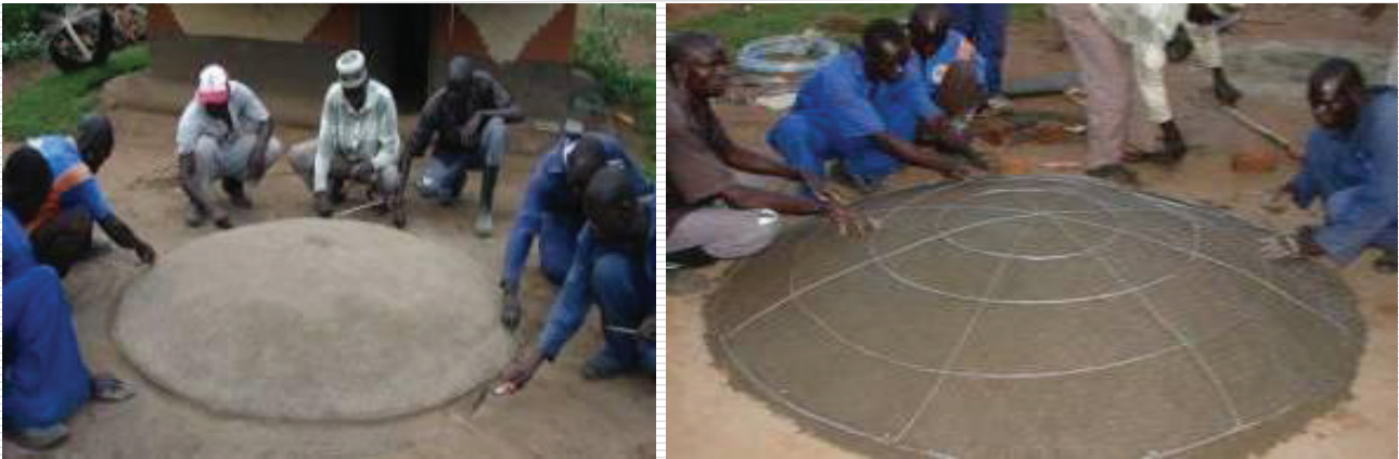
Figure 15: Dome made of compacted soil for cover mould (left) and reinforcement wires placed over chicken mesh.
