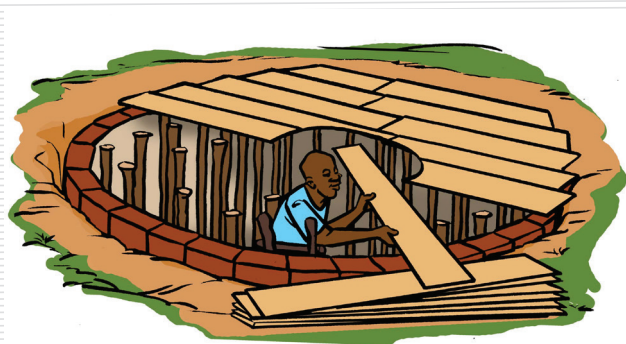
Figure 25: Lay horizontal pieces of timber at the spacing of 1 m parallel the mouth of the tank
