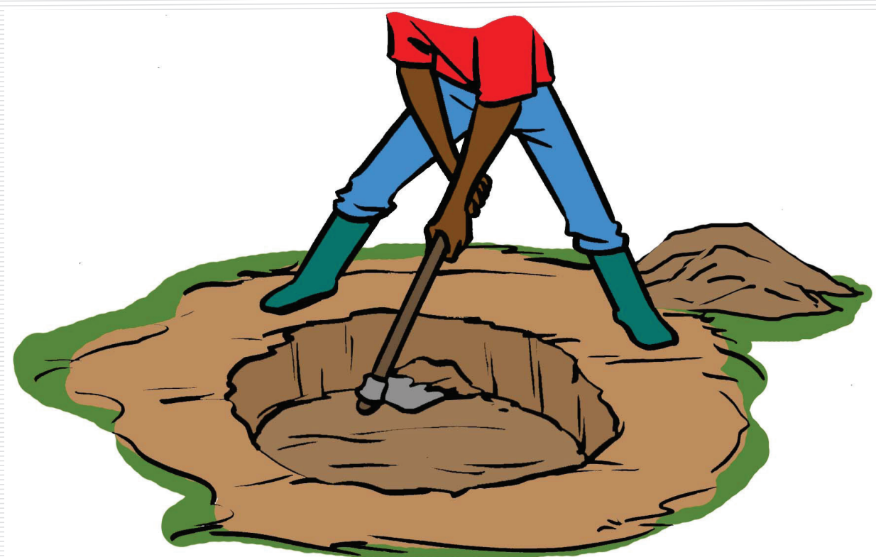
Figure 40: Excavate up to 1m below the ground
