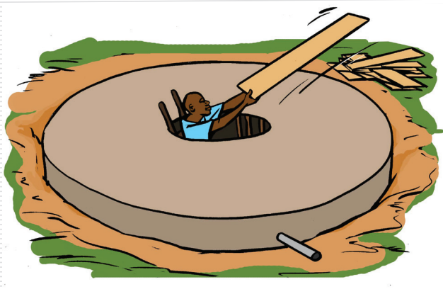
Figure 28: Removing the shutters
