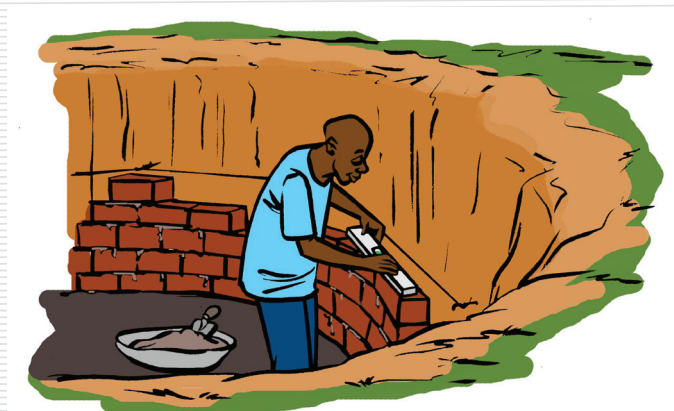
Figure 23: Use of a spirit level ensures accurate vertical and horizontal levels
