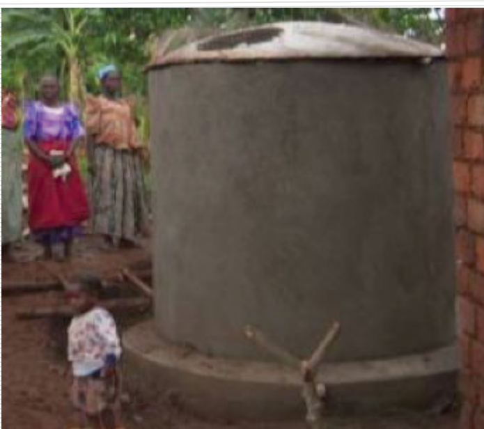
Figure 16: Tank cover in position ready for finishing coats
