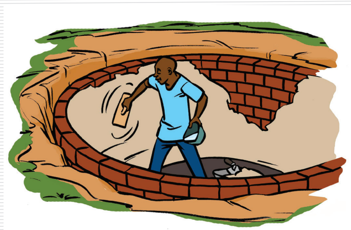
Figure 24: Plastering the inside of the tank
