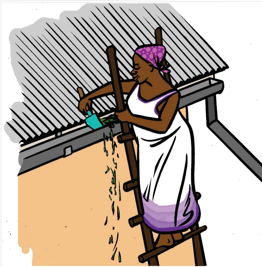
Figure 10: Gutters and covers should be cleaned periodically after leaf fall
