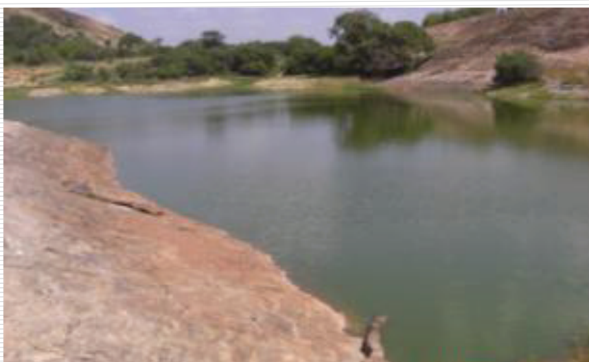
Figure 36: Large dammed storage for a rock catchment system
