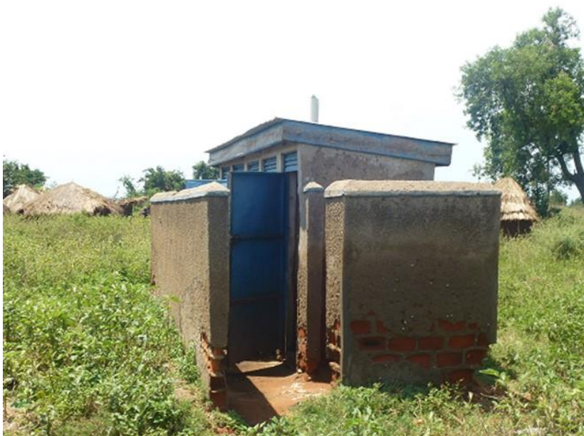
Plate 6-2: Community Pit latrine that will be affected by the Transmission Line
