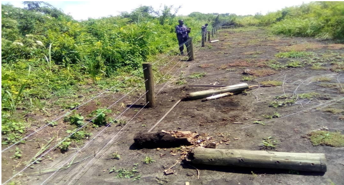
Plate 5: Examples of gum fence poles being replaced at MFCA at the moment
