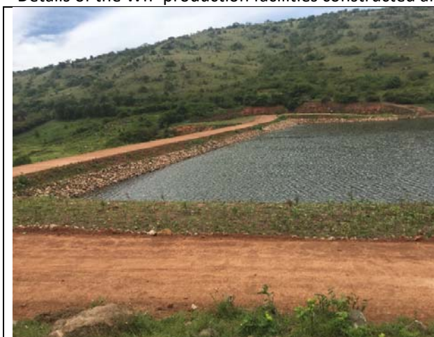
Photo 7-2-1 Current status of Kagango dam in Isingiro District.
