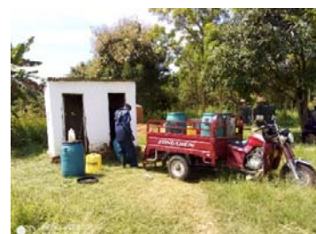
Photo 7.1.4-3 Emptying of the toilet by gulpers (left) and loading of sludge on Tri cycle (right)
