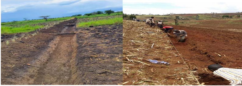
Photo 3-2: Infiltration trenches constructed in Aswa catchment (Left) and Awoja catchment (Right)
