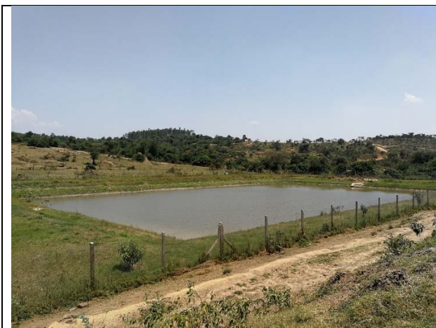
Photo 7-2-5: Katongole Communal valley tank in Mubende District
