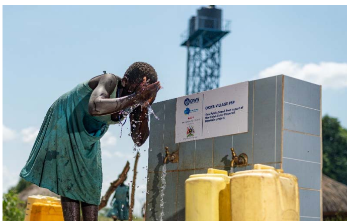
Photo 8-1 piped water supply by CSO
