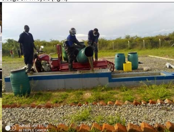
Photo 7.1.4-5 Disposal of faecal sludge at Dzaipi FSTP, by gulpers
