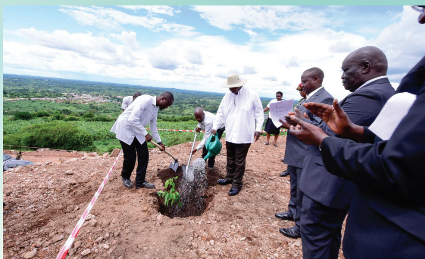
HE President planting a tree during the ground breaking of Kikyenyeky-Nabuhiky GFS in Ibanda district as the Ministry officials look on
