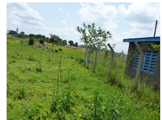
Busolwe mini water reservoir in a seasonally flooded grassland located along Busolwe – Tororo road
