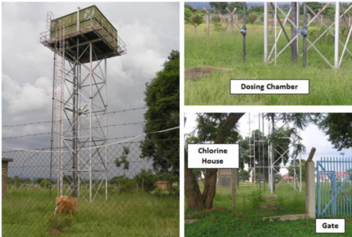
Photo 2: Existing reservoir structures at Budaka
