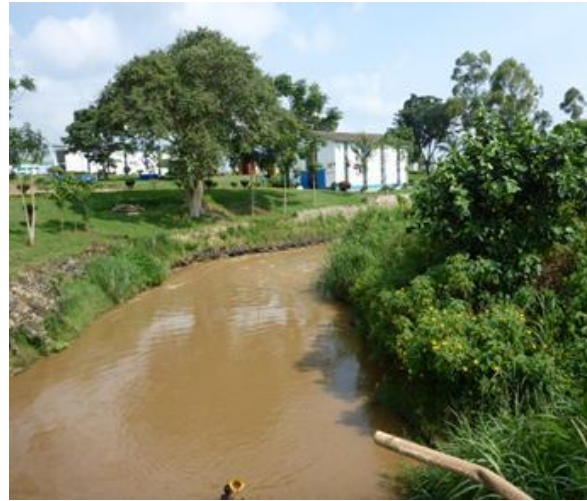
Photo 4: Manafwa river and treatment plant
