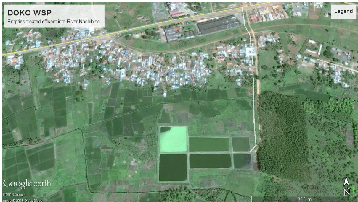
Figure 54 Doko Waste Stabilization Pond which empties into R. Nashibiso
