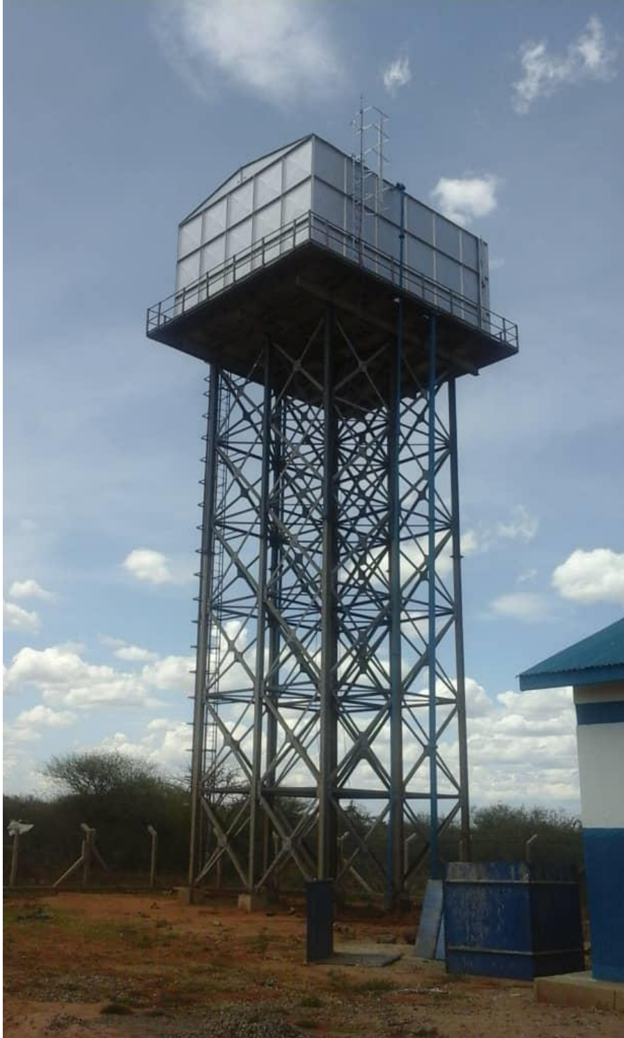
Amudat reservoir with a capacity of 150m 3 on a 15m steel tower
