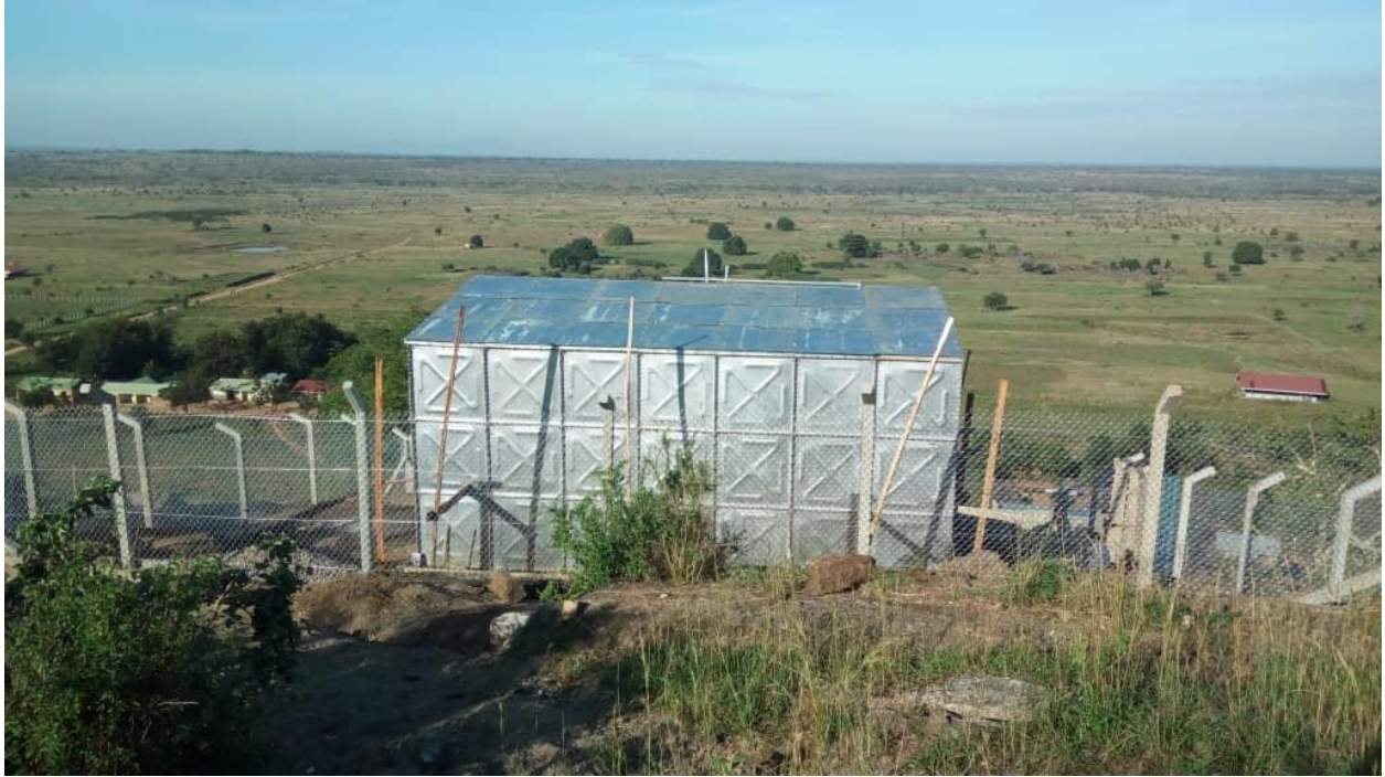
Kacheri water tank capacity of 156\text{m}^3 steel reservoir on an elevation of
