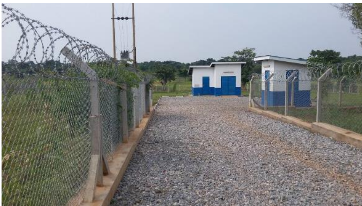
Plate 1-3: Existing pump station in Kaliro town
