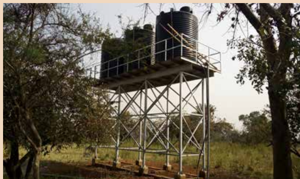
Storage in overhead tanks for irrigation
