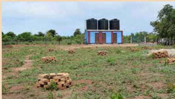
Water Storage tanks for irrigating the gardens
