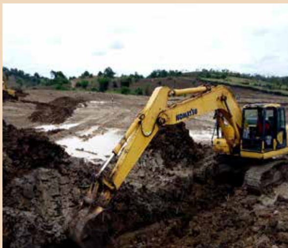
Excavation of an inlet for a valley tank in Kyegegwa District
