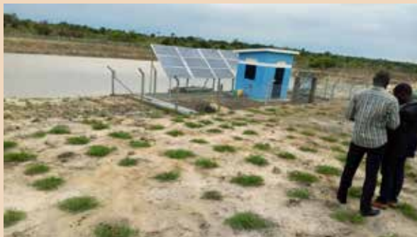
Water source and Abstraction system
