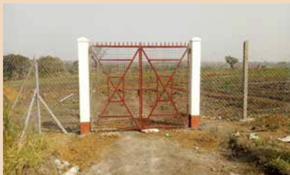
Fenced irrigation system to provide security
