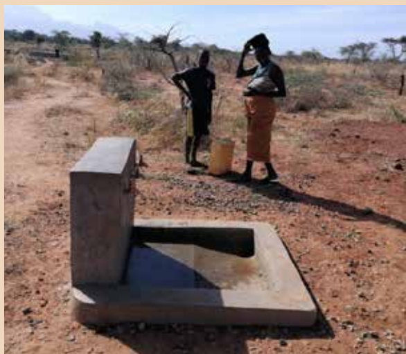
Tap stand with three (3) taps was functional
