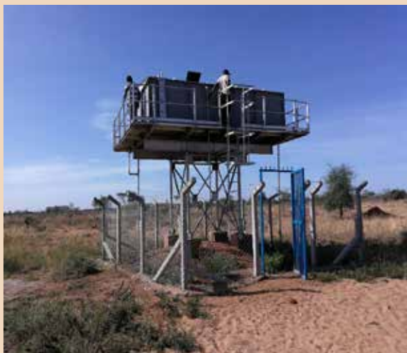
Reservoir was functional with no leakages observed
