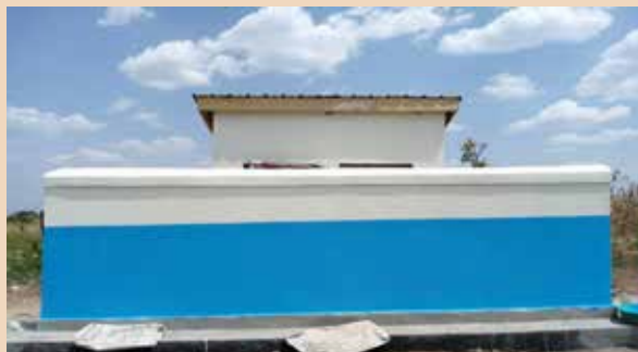
Completed lined VIP latrine at Opwach SSIS
