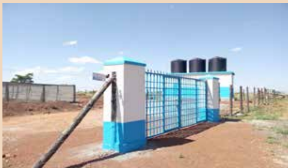
Fencing of the irrigation systems at Opwach completed
