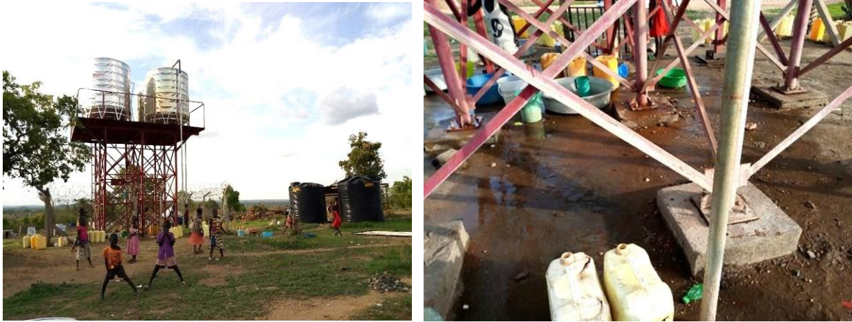
Figure 6-4: Water spillage at a storage tank in Rhino Camp Settlement.
