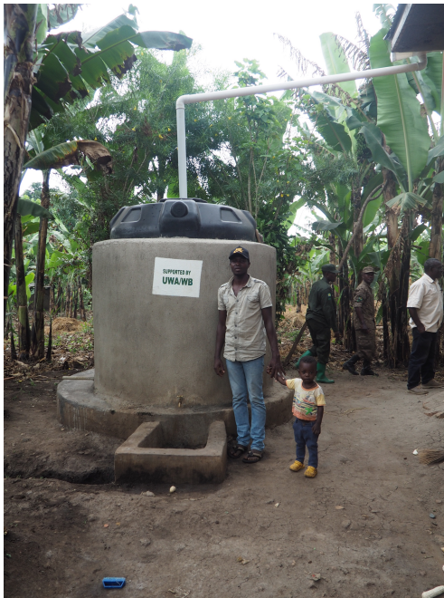
Installation of water tanks requires a metal roof, guttering and fascia board
