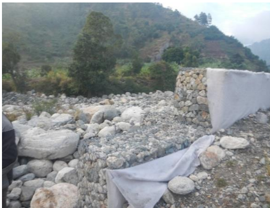
Figure 4-5: Gabion walls to attenuate River Nyamwamba floods at perilous hotspots in Kilembe Subcounty
