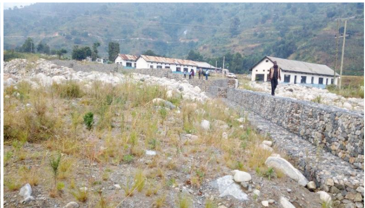
Figure 4-5: Gabion walls to attenuate River Nyamwamba floods at perilous hotspots in Kilembe Subcounty
