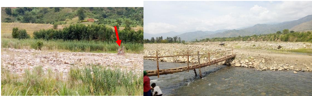
Figure 4-6: Makeshift bridges used for crossing the River Nyamwamba
