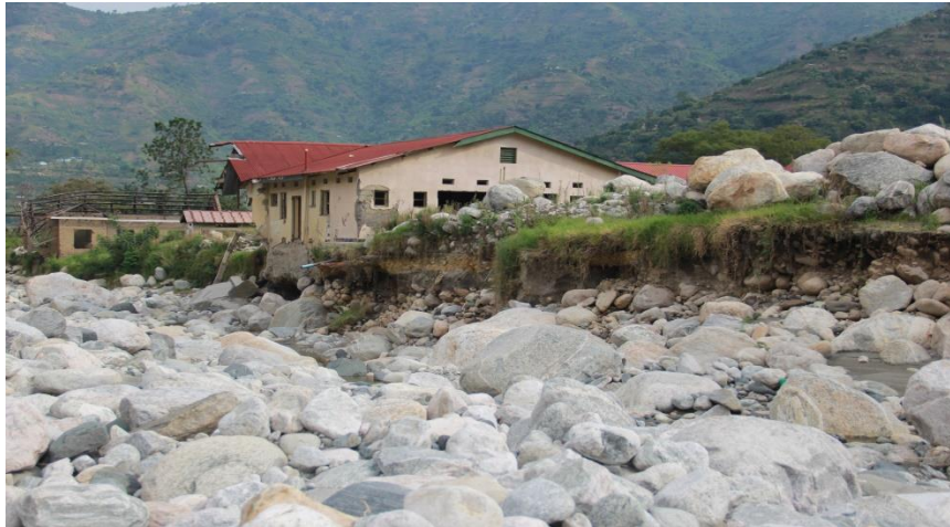
Figure 5-12: Kilembe hospital damaged during flooding
