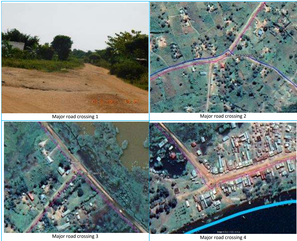
Figure 2-13: Major Road crossings by the transmission and distribution pipelines in Lugala RGC
