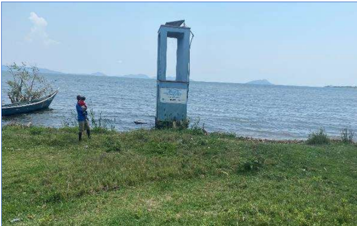
Figure 2-3: Raw water abstraction point for Lugala Centre RGC
