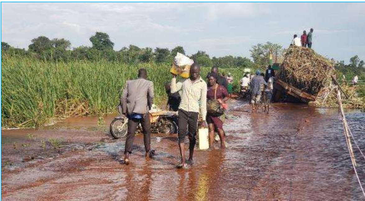
Figure 6-19: Flooded bridge under construction along Lumbuye wetland in Matete Village
