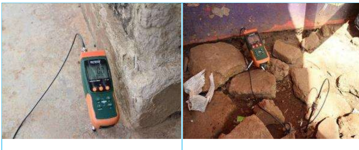
Figure 2-4: Field measurements for vibrations
