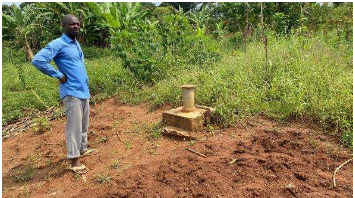
Figure 3-3: Drilled borehole for Bukizibu-Bumwena RGC
