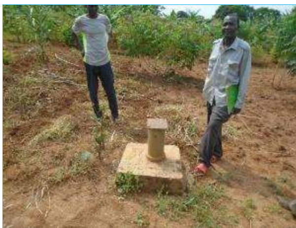
Borehole Water Source in Malongo Sub-county; 36 N 0556693, 0029165
