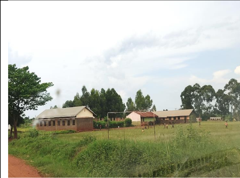
Mboira Trading Centre and Primary School (E 378989, N 202683)
