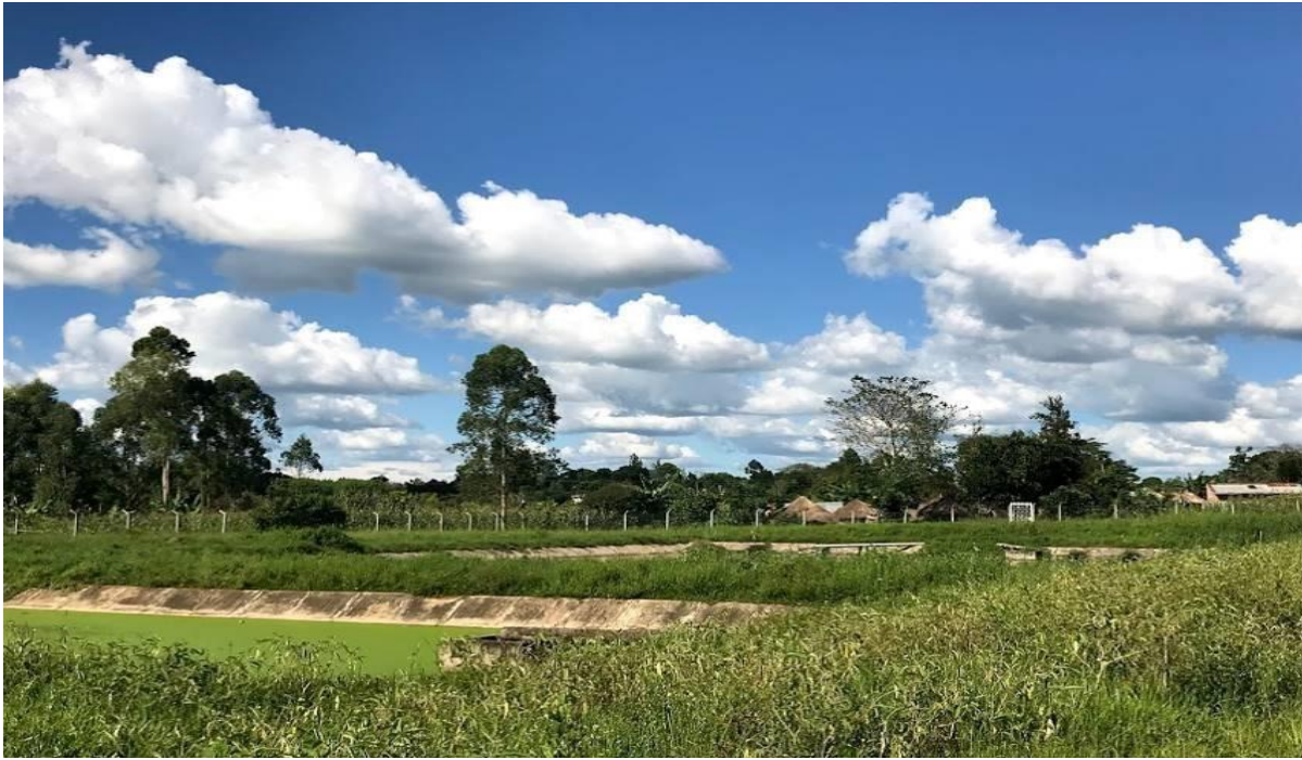
Figure 7-3: Waste Stabilization Ponds at Kiryandongo Hospital
