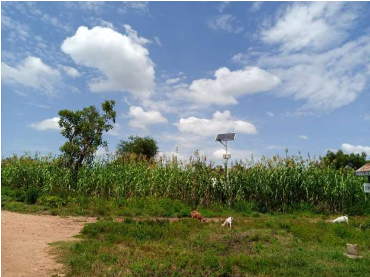
Plate 5.15: One of the public solar lighting systems
