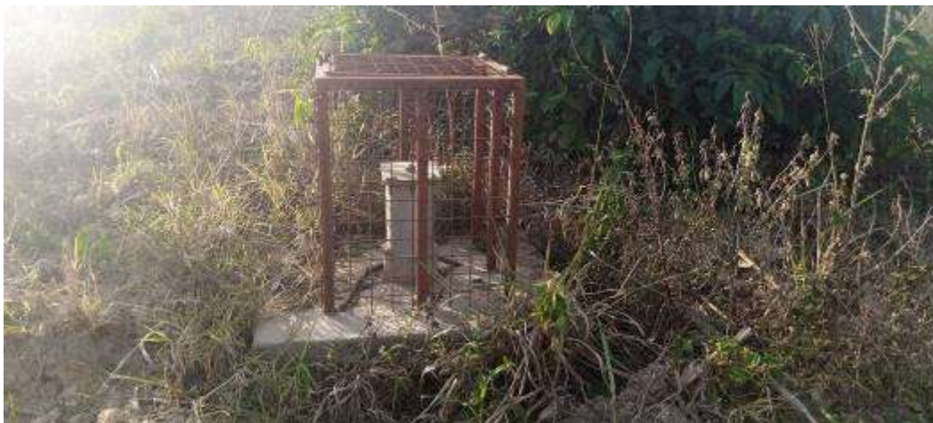
Plate 1: The drilled borehole as the potential water source
