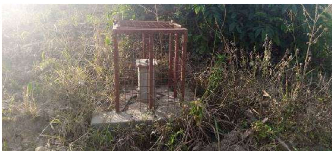
Plate 6: Mwitanzige water supply production well.
