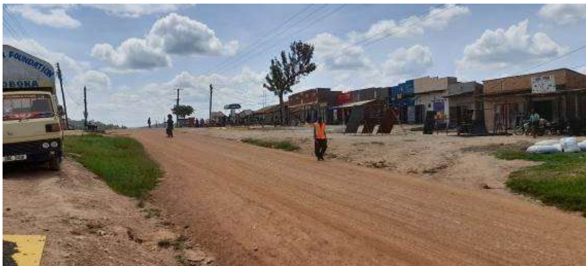
Plate 9: The Lyantonde-Rakai Road through Lwentulege Town Council
