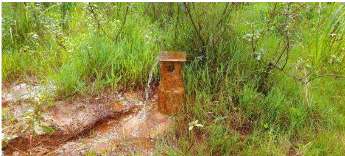
Plate 6: Lwentulege water supply production well.
