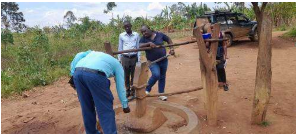
Plate 8: One of the handpump borehole in the project area that almost dries up during dry season
