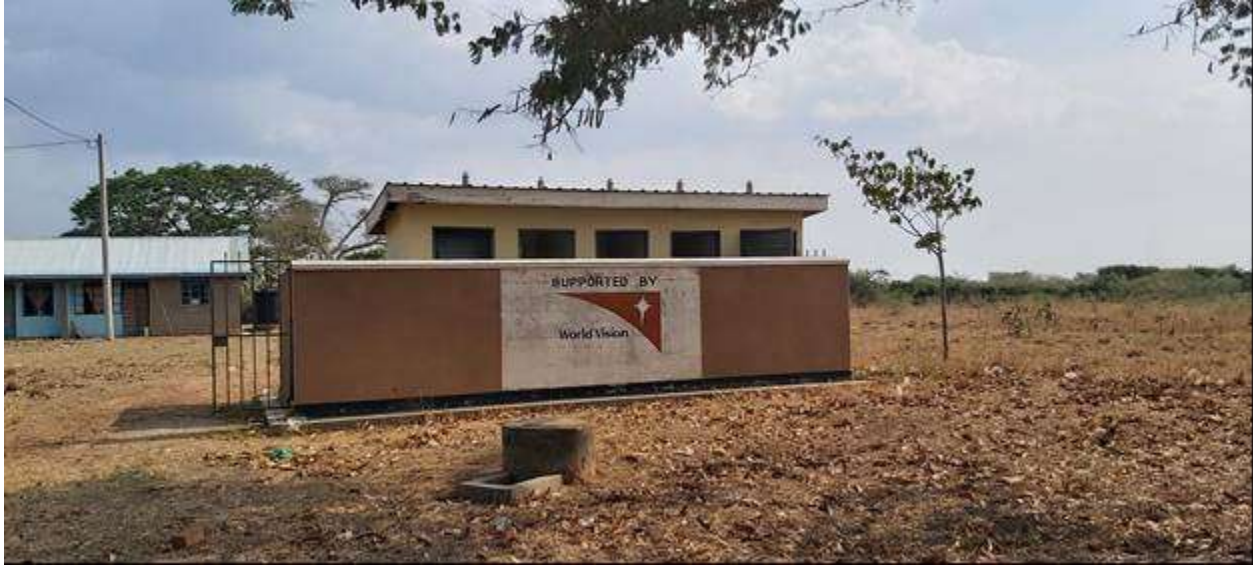
Figure 5-51: Public Toilets constructed by World Vision in Kikooge Rural Growth Center.
