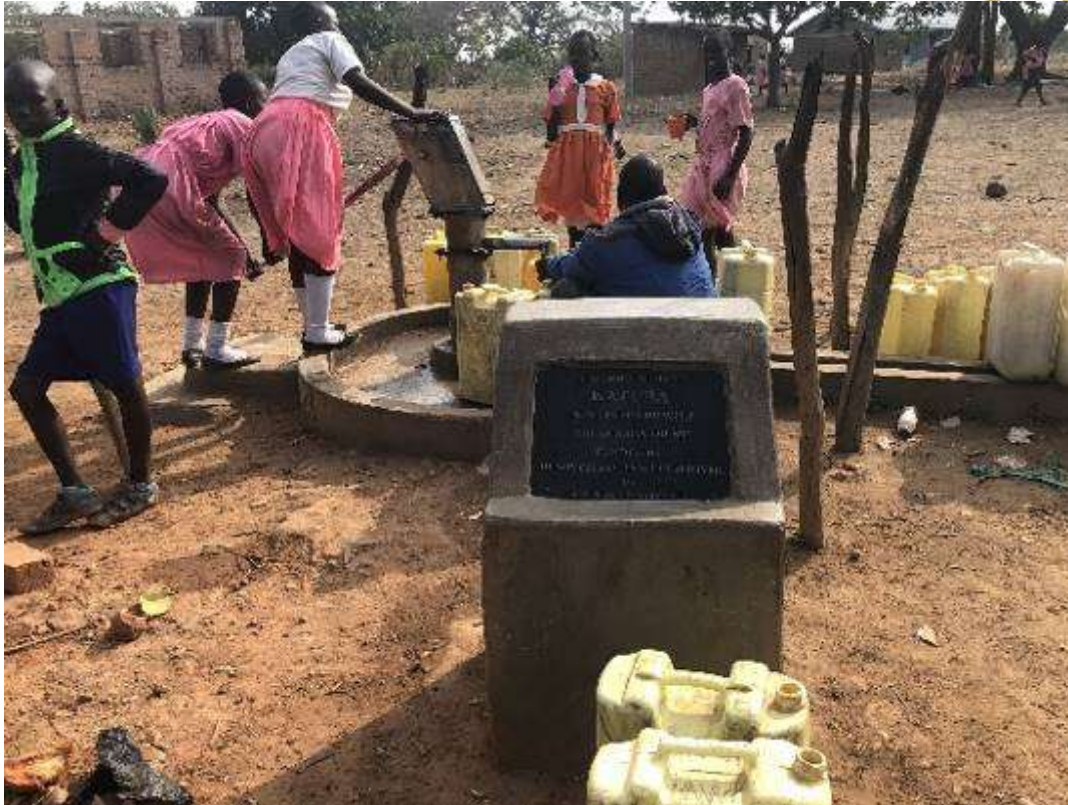
Photo 5-4, Borehole at Katuba at 36N 418962 177139
