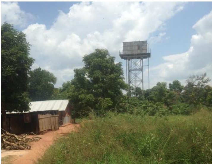
Photo 2: Existing elevated tank in Kamdini
