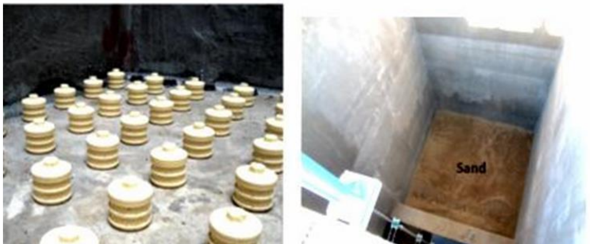
Photo 4: Nozzles at bottom of filter (left), and filter filled with sand (right)
