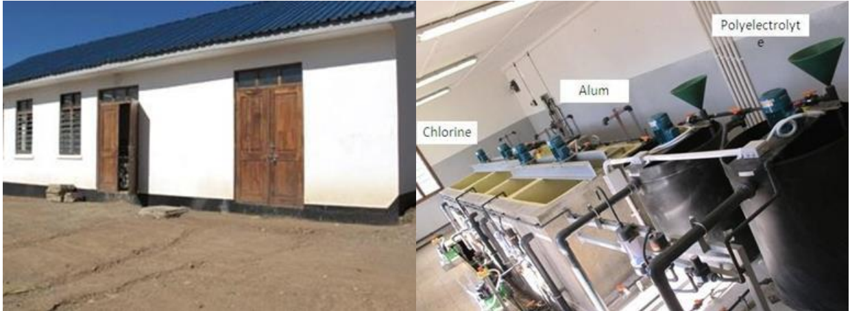
Photo 5: Typical chemical dosing building
