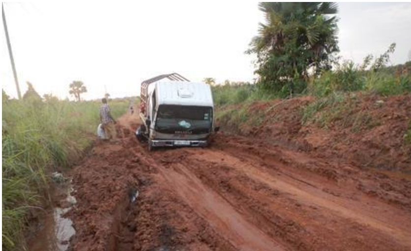
Photo 55: State of one of the community roads after a heavy rain
