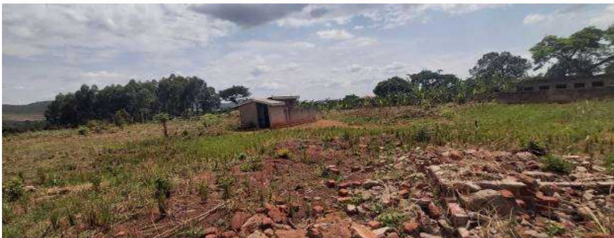
Figure 5-16: VIP pit latrines at Bugomolwa Primary School.
