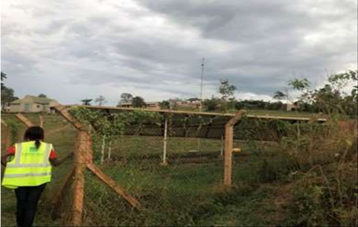
Photo 5-10 Solar motorized borehole construction in JICA at Lubaali Rural Growth Center.
