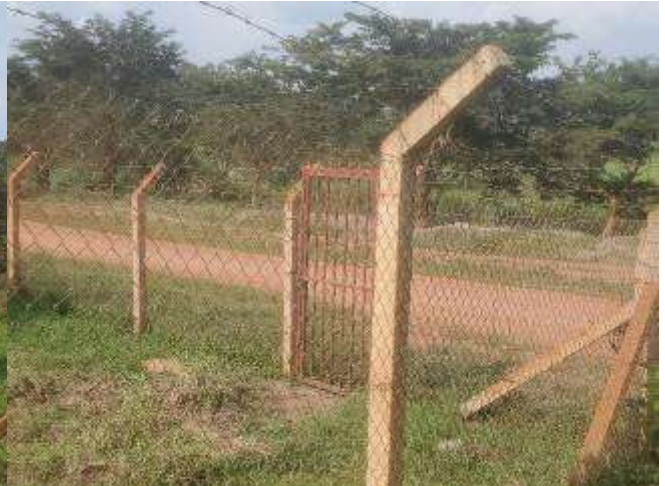
The access road and the source fencing
