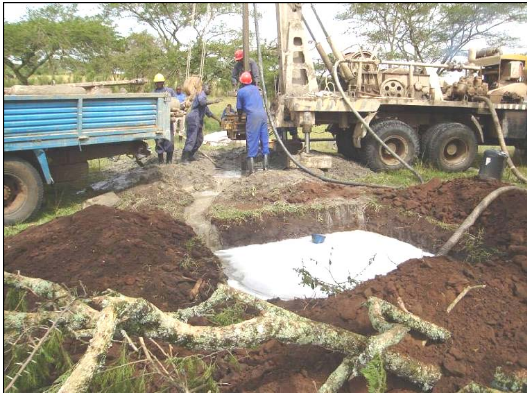
Figure 4: Illustration of mud drilling and the location of the mud pit
