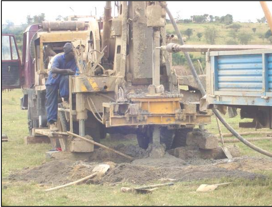
Figure 5: Air percussion drilling.
