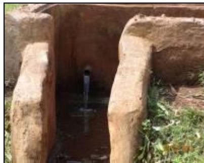
Protected Spring in the Catchment
