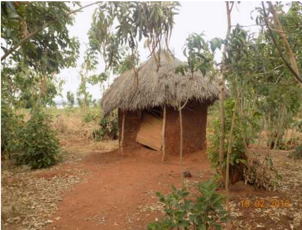
Picture 4-5: Example of pit latrines in project area
