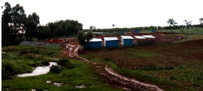
Construction site where treatment plant is located
