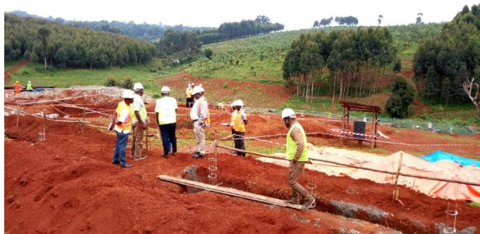
MWE team inspecting the construction site construction of Reservoir tank
