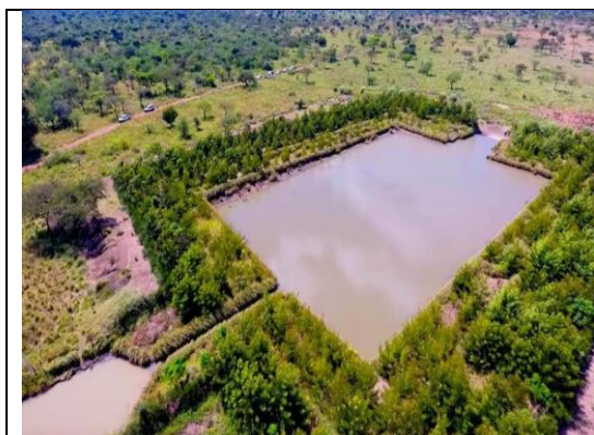
Photo 7.2-1: A well protected Loho Valley Tank in Kacheri Sub-county, Kotido District
