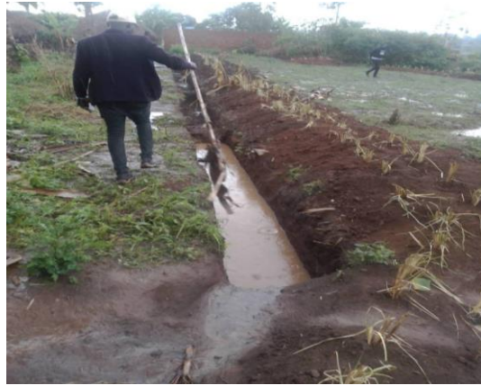
Photo 3-2: Soil and Water conservation structures established in Aswa II sub-catchment
