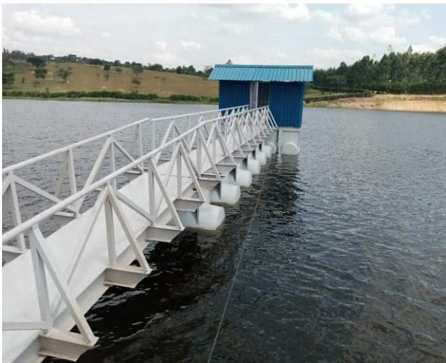
Photo 1: Kyenshama earth dam in Mbarara District under construction.
