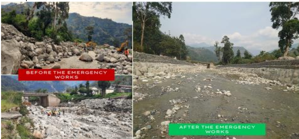
Photo 3-8: Emergency maintenance works for R. Nyamwamba
