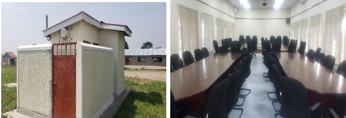
Photo 3-5: Completed Toilet block and Conference Hall
