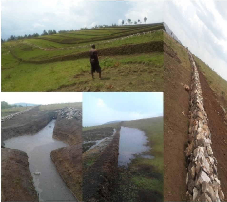
Plate 10: Some of the measures implemented in Mashyoro Micro catchment: stone bunds (top and right) and infiltration pits (bottom left)
