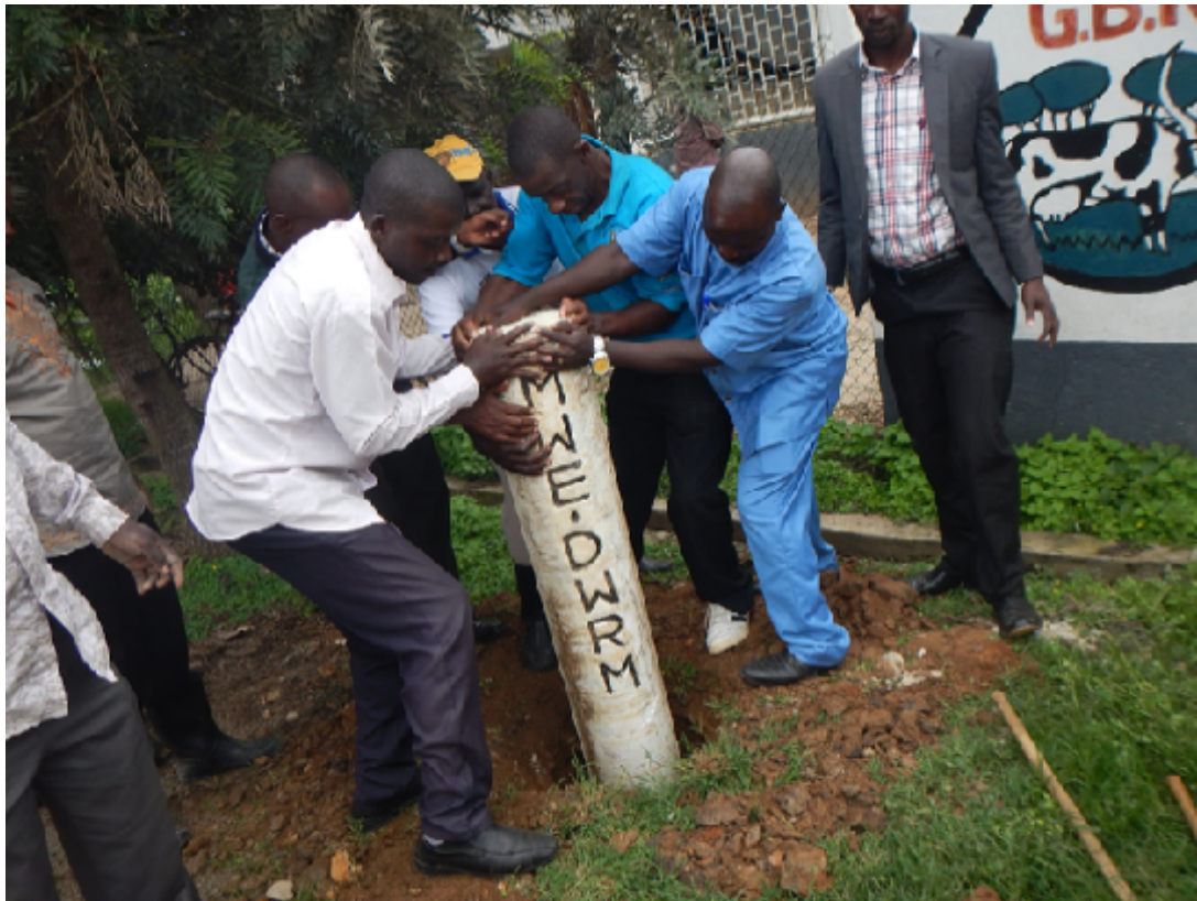
Plate 13: Installing a boundary pillar near GBK premises
