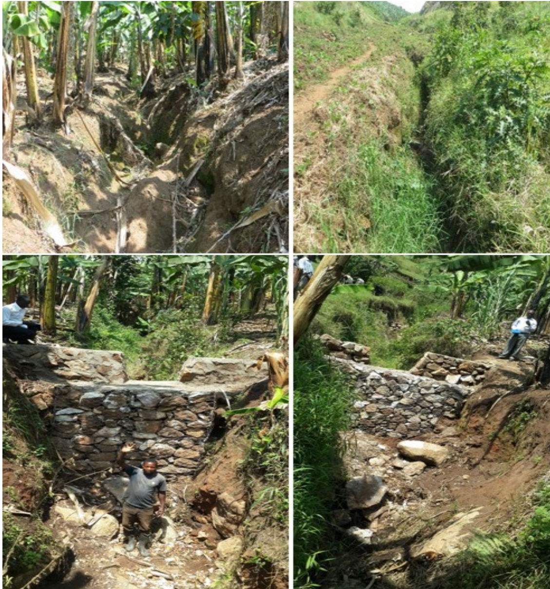
Plate 9: Gullies (Top) and check dams (bottom) constructed in gullies to regulate water flow and trap debris from upstream
