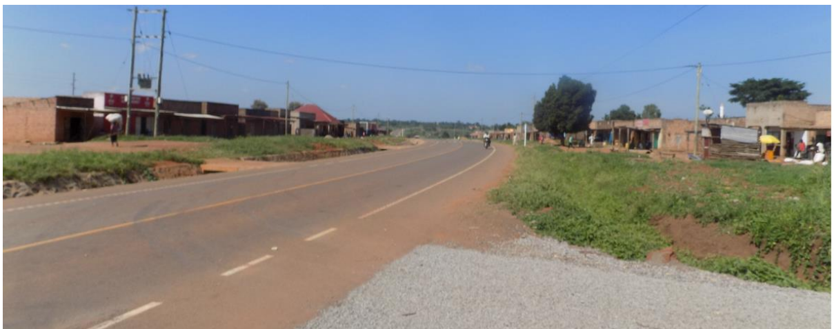
Figure 5-22: Nyakabale Trading Centre along Kigumba - Masindi Road
