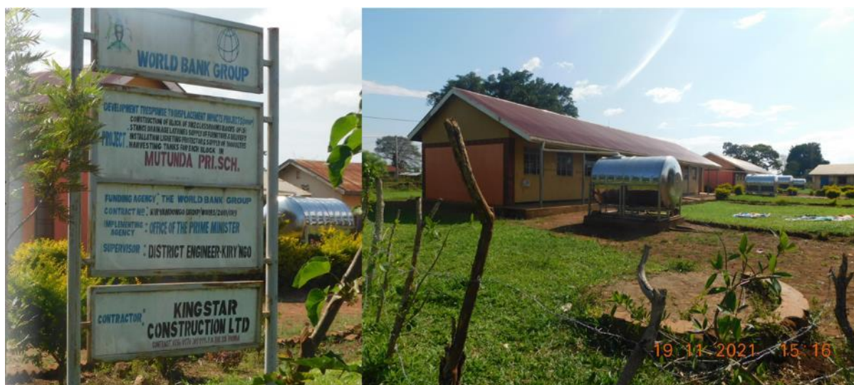
Figure 0-70: Steel water tanks at Mutunda primary School
