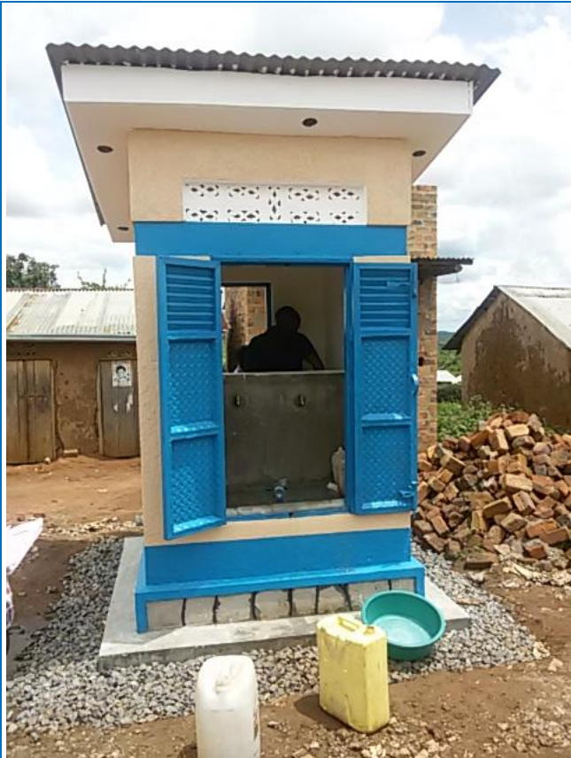
Public Water Kiosks; Two hundred forty-nine (249) units were constructed.
