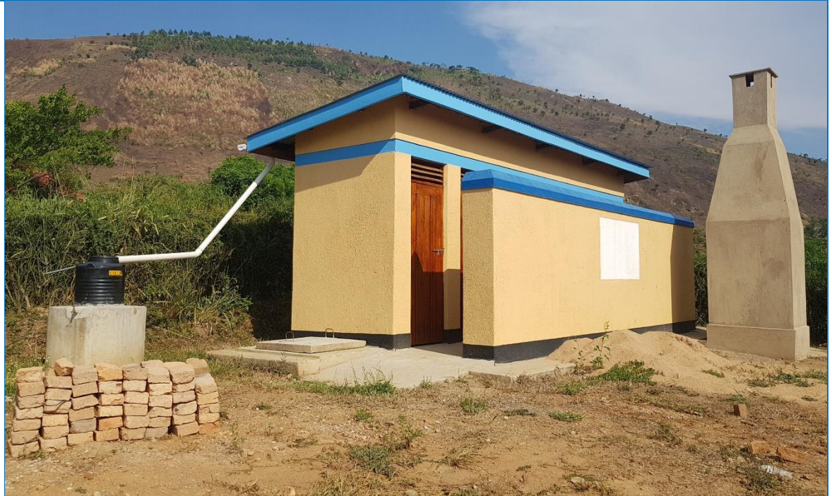
Institutional toilets: Eight (08) Lined-pit latrines were constructed to completion.
