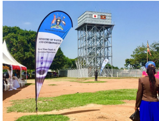
MWE in collaboration with JICA for improved Water Supply and Sanitation in the selected Rural Growth Centers Eastern Uganda at Kibuuku District.
